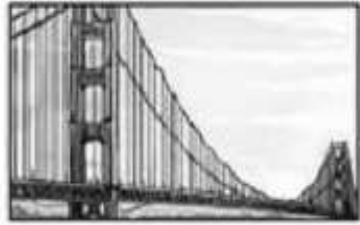
Picture 11. golden gate bridge
